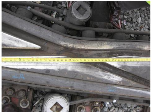
Figure 8: "Blip" and Ramp on D2
