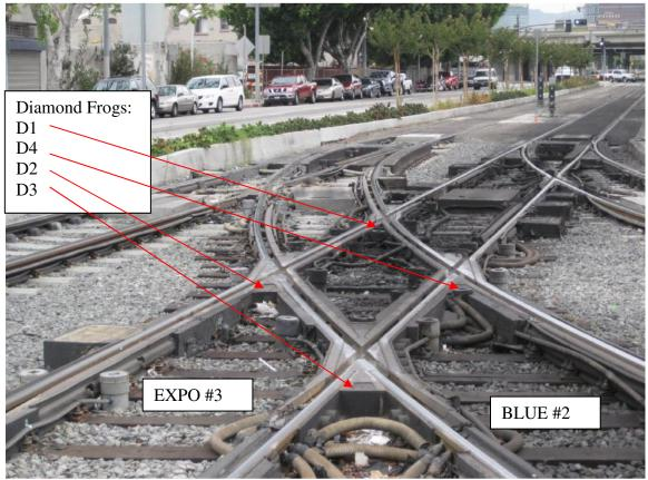
Note: RED arrows indicate direction of normal travel. Figure 1: Junction with all four Diamond Frogs (D1-D4)
