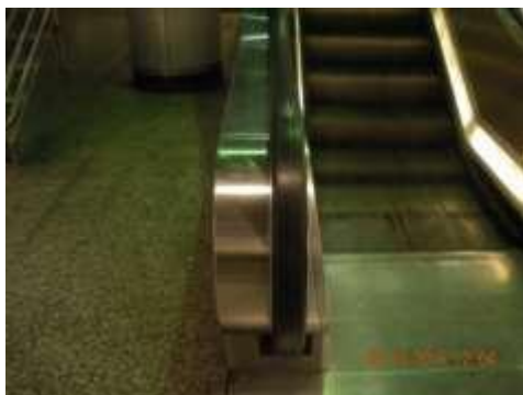
Missing caution decal on left side of escalator
