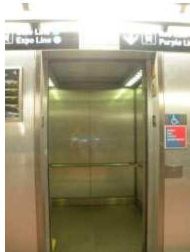
7 th St/Metro Center Station Missing In Case of Fire sign on elevator
