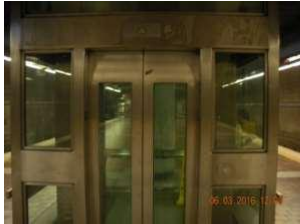
7 th St/Metro Center Station Missing all 4 signs on elevator
