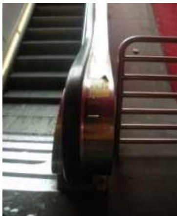
Westlake/MacArthur Park Station Peeling caution sign decal on escalator
