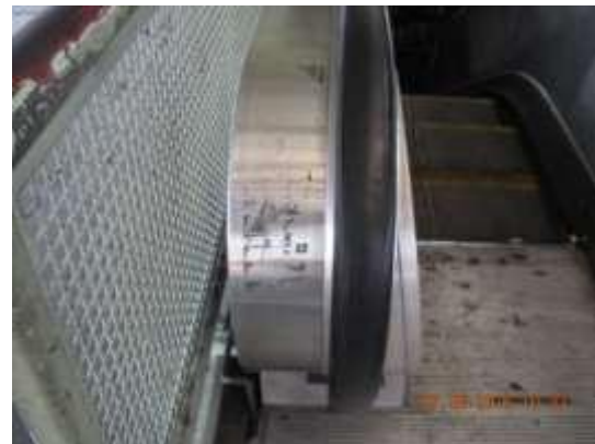
Willowbrook/Rosa Parks Station Missing caution decal
