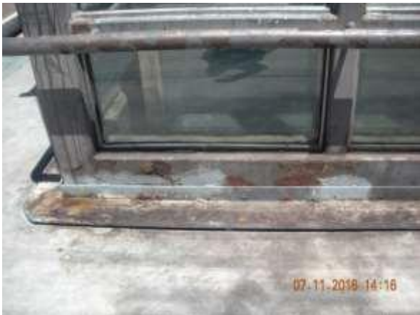
Avalon Station-Green Line Rust on Elevator #L5W
