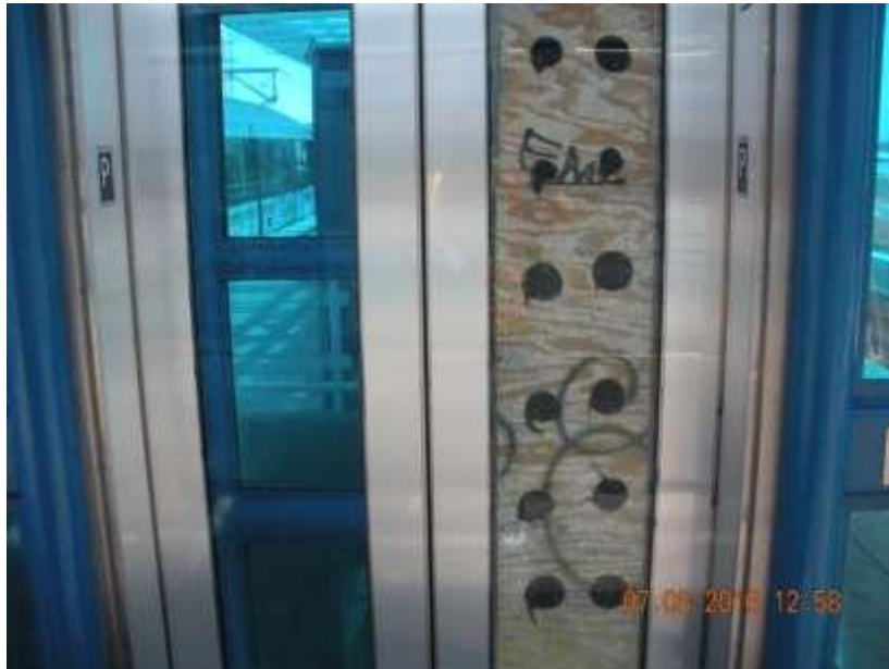
Redondo Beach Station-Green Line Elevator #L-1822 Broken glass door window covered with wood that has graffiti on it
