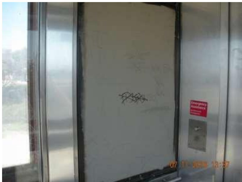
Vermont/Athens Station-Green Line Elevator #L3W Broken glass window covered with wood
