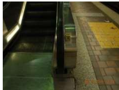
Missing caution and call decals on right side of escalator
