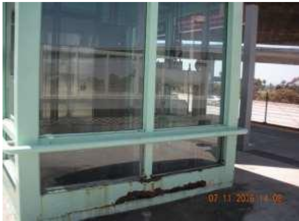
Harbor Fwy Station-Green Line Rust on Elevator #L4E
