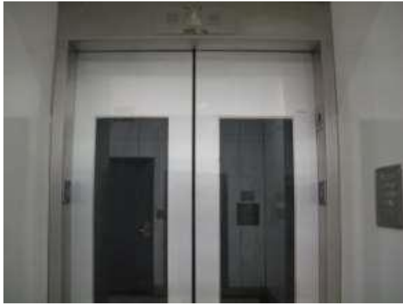
Pershing Square Station-Red/Purple Line Missing Star of Life signs on elevator
