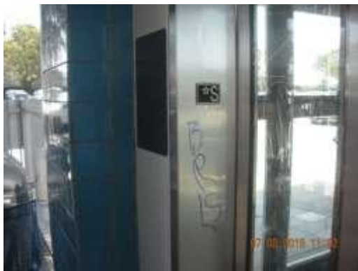
Del Amo Station-Blue Line Graffiti on Door of elevator #DEL-01
