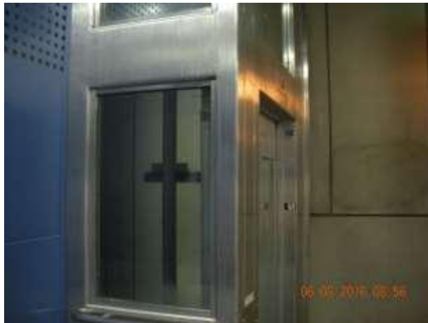
Vermont/Sunset Station-Red Line Missing handicap sign on elevator
