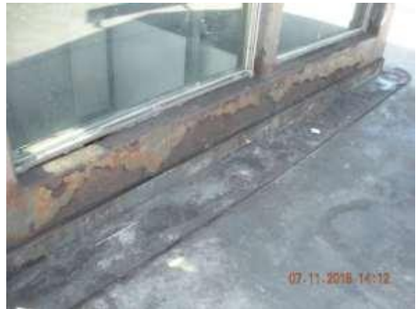
Avalon Station-Green Line Rust on Elevator #L5E
