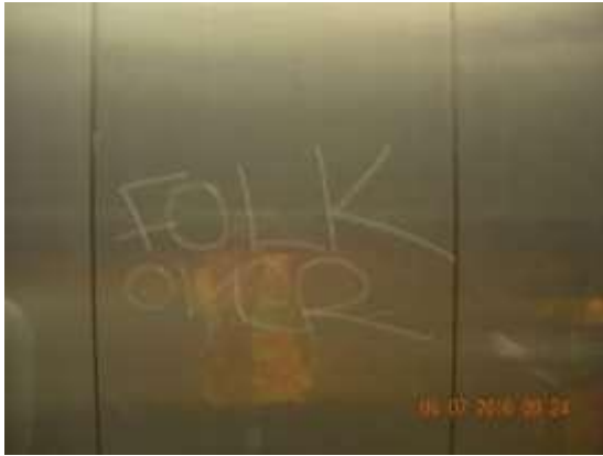
MacArthur Park Station-Red/Purple Line Graffiti on side of escalator #503
