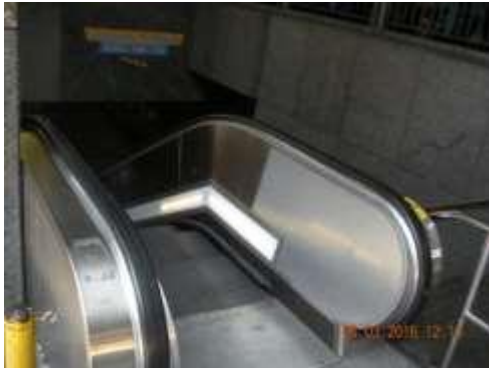
7 th St/Metro Center Station Missing caution sign on left side of escalator
