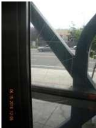
La Cienega Station-Expo Line Graffiti on glass window of elevator #LC-2
