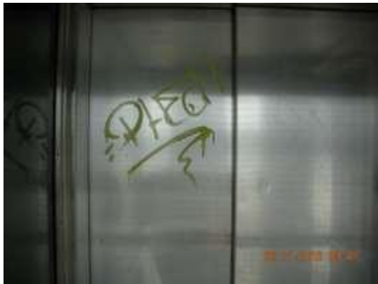
Lake Station-Gold Line Graffiti inside on door of elevator #LS-1
