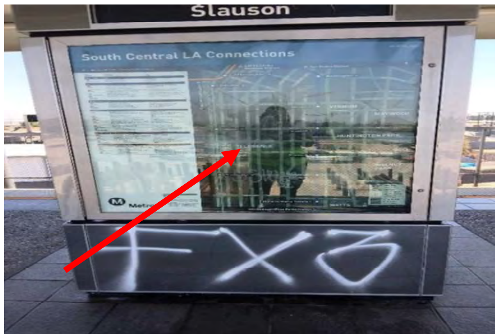
Slauson Station: 2024A-006 July 30, 2025 - Damaged Map Case
