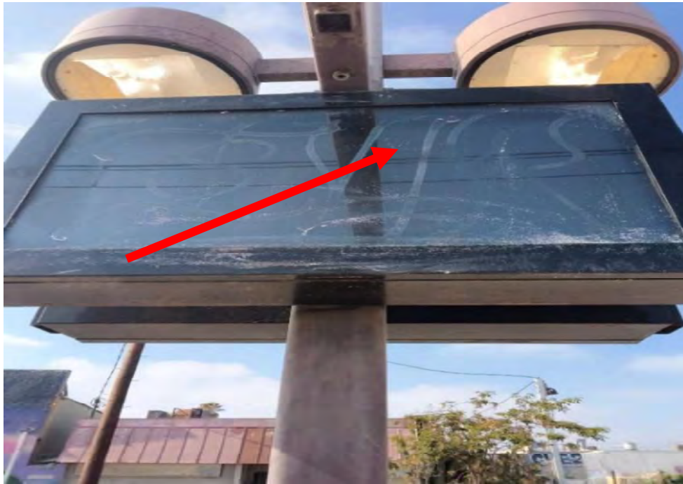
Pico/Aliso Station: 2024E-001 July 29, 2025 - Broken Monitor
