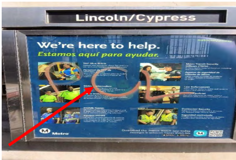
Lincoln/Cypress Station: 2024A-004 July 30, 2025 - Graffiti
