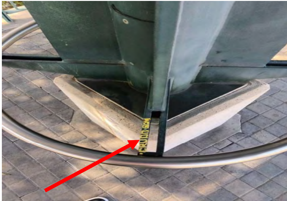
Lincoln/Cypress Station: 2024A-002 July 30, 2025 - Graffiti
