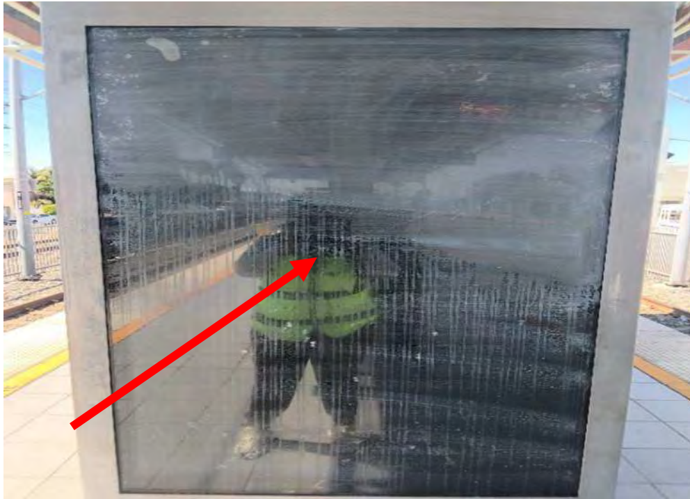
Compton Station: 2024A-007 July 30, 2025 - Damaged Map Case
