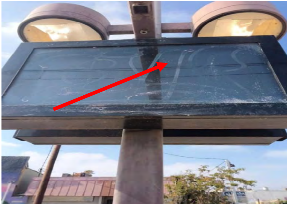
Pico/Aliso Station: 2024E-001 July 29, 2025 - Broken Monitor
